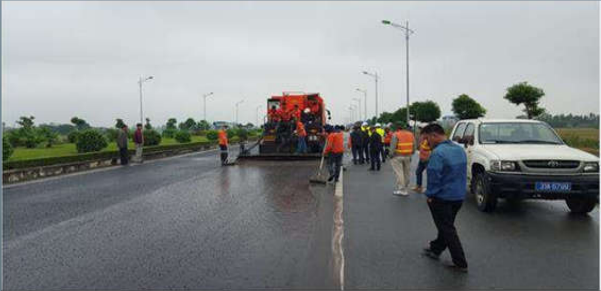
TRIAL CONSTRUCTION AT NATIONAL HIGHWAY 21B – HAI PHONG
