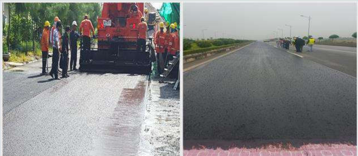
TRIAL CONSTRUCTION AT NATIONAL HIGHWAY 5 – HAI PHONG
