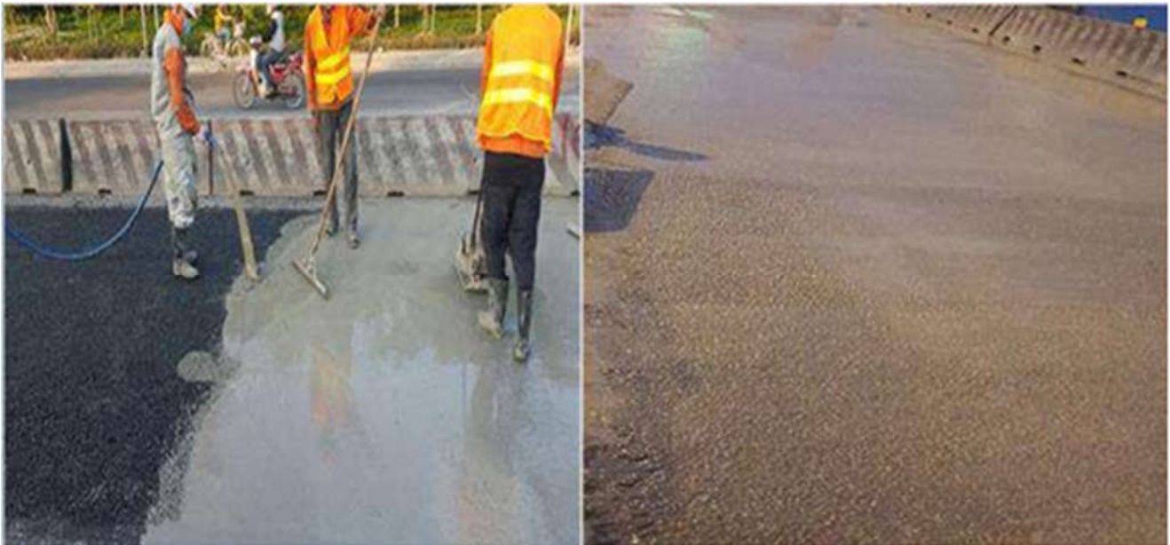
Semi-flexible pavement National Highway A1 (An Suong – An Lac segment)
